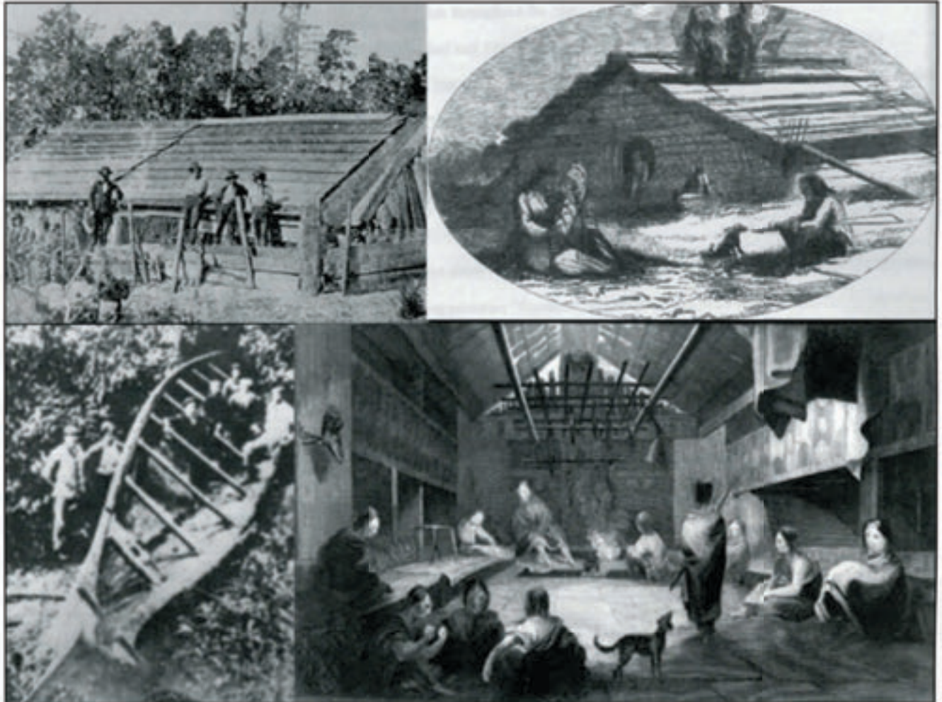
Figure 2. Precontact large-wood products. Upper Right: Traditional Kelawatset (“Quuiich”) cedar plank house photographed by an Army officer near mouth of Umpqua River in 1858; Upper Right: Drawing of a similar plank house near the same location, published by Harper’s Magazine, also in 1858; Lower Left: Large sea-going trade canoe found near mouth of the Salmon River in Lincoln County; Lower Right: Interior of typical Chinookan lodge along the Columbia River, drawn by Alfred Agate in 1841.
